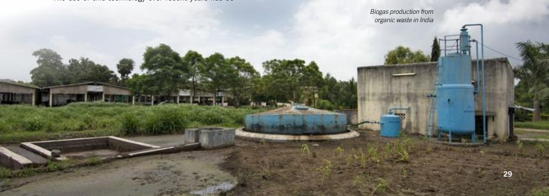
As a rule, roughly 10 kg of kitchen and market waste are needed to produce  $1-1.5\ \text{m}^3$  of biogas. This amount of biogas contains approximately 6 kWh of energy which substitutes  $0.5\ \text{l}$  of diesel fuel.
