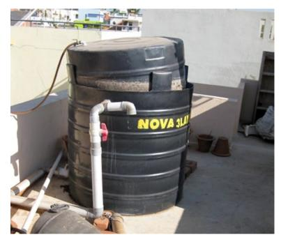
Producing biogas in a domestic digester
