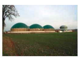
Waste digestation plant (1  $MW_{el}$ ) with an input of 24,000 t per year
