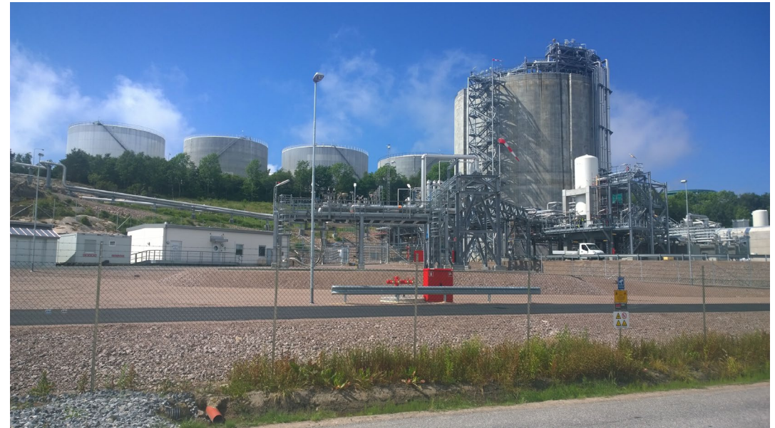
Lysekil terminal in Sweden
